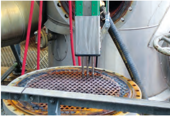
Cleaning the inside of the heat exchanger
