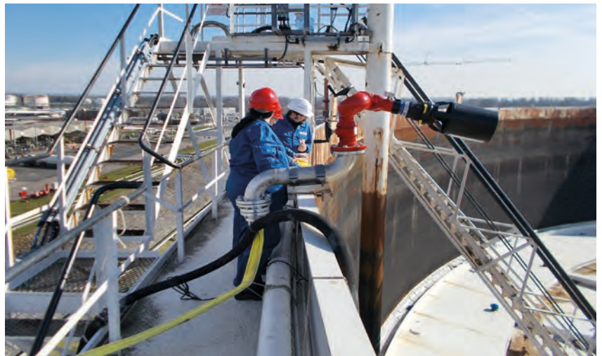
Visually inspecting the BTS Blabo® jet washer system
