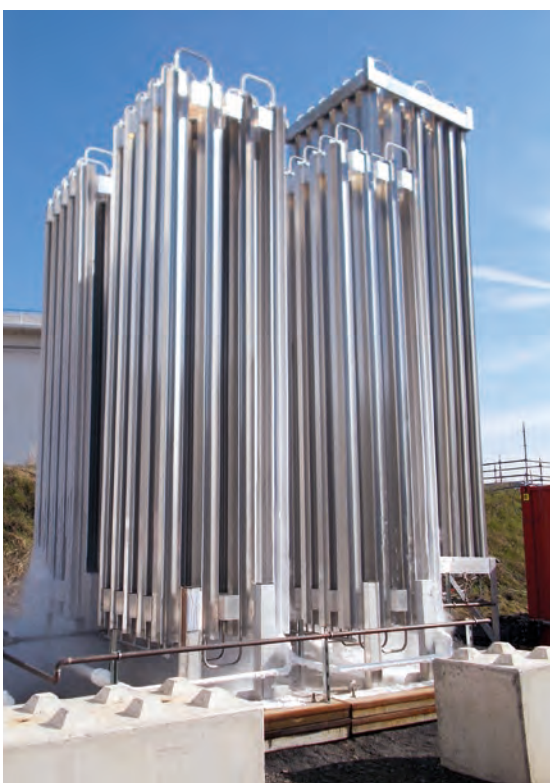
The nitrogen evaporator used to create an inert atmosphere in the tank
