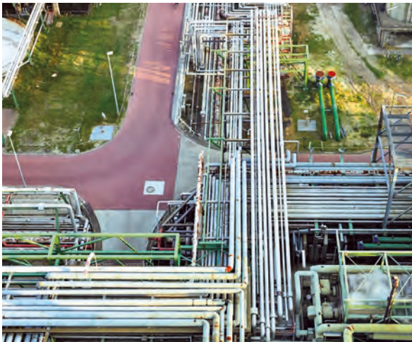
The pipes leading to the crude oil distillation facility in Lingen
